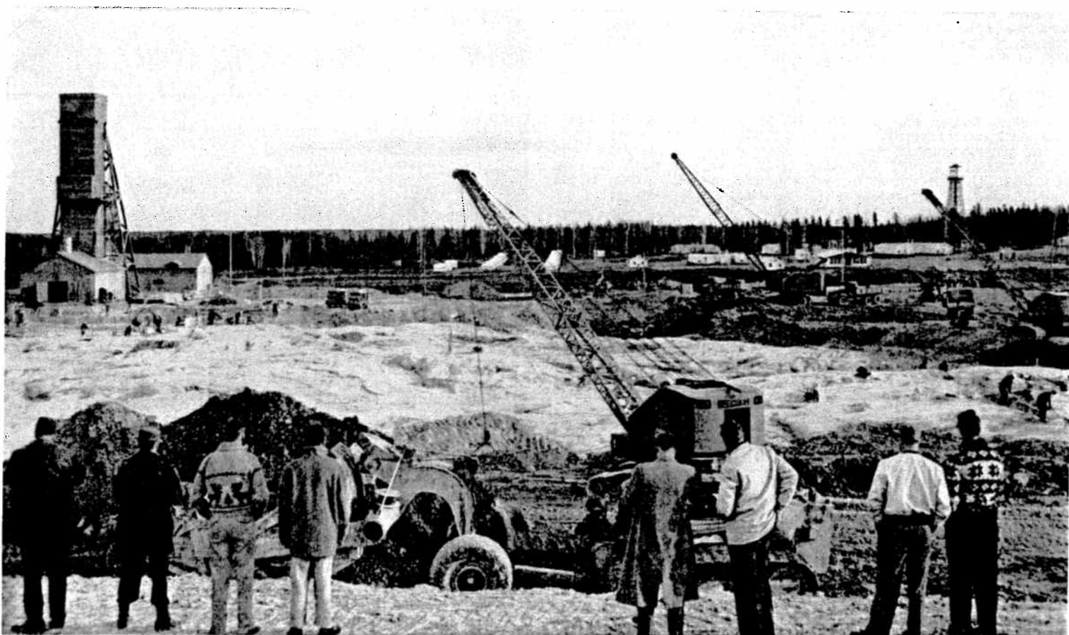
The plant area at Thompson was a scene of great activity as powerful earth-moving equipment cleared the site for the 9,000-ton concentrator. The smelter will stand on ground immediately to the right of the picture. In the left background is the temporary headframe of the Thompson mine production shaft.
