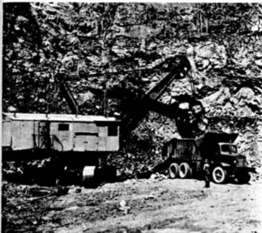
One of the Open Pit's huge electric shovels is seen in this closeup, filling a haulage truck with its 30-ton load. The shovel is equipped with four motors with a total capacity of 250 hp., has a bucket capacity of 4\frac{1}{2} yards, weighs in all 170 tons. The truck has a 275 hp. diesel motor, weighs 60 tons when loaded. Bulldozers and graders maintain the roads into the pit and are constantly engaged in a "good housekeeping" program on the pit bottom.
