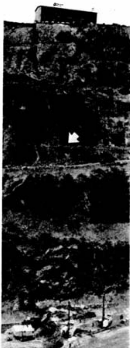
In this unusual view at the Open Pit, the crushing plant is seen at the top while, 500 feet down, a shovel and two churn drills work on a new bench. Midway, indicated by the white arrow, is a timbered drift which has been driven into the footwall. From it longhole drilling has been fanned out with the objective of cleaning off recovery ore (darker in color) from the footwall. This particular program is an indication of the thorough manner in which the Open Pit is being mined.
